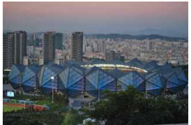
Main Stadium of Universiade Center
